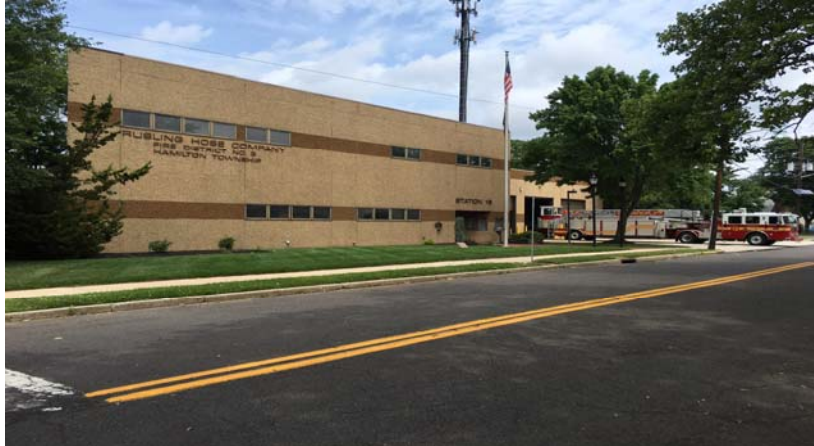
Fire District No. 3, Rusling Hose Fire Company, Station 13, 13 Rennie Street
