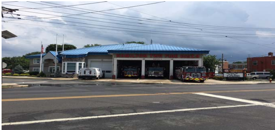
Fire District No. 4, Hamilton Fire Company, Station 14, 1805 East State Street
